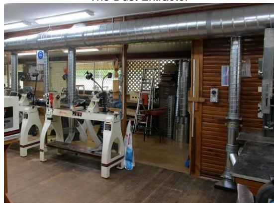
Some of the Ducting
